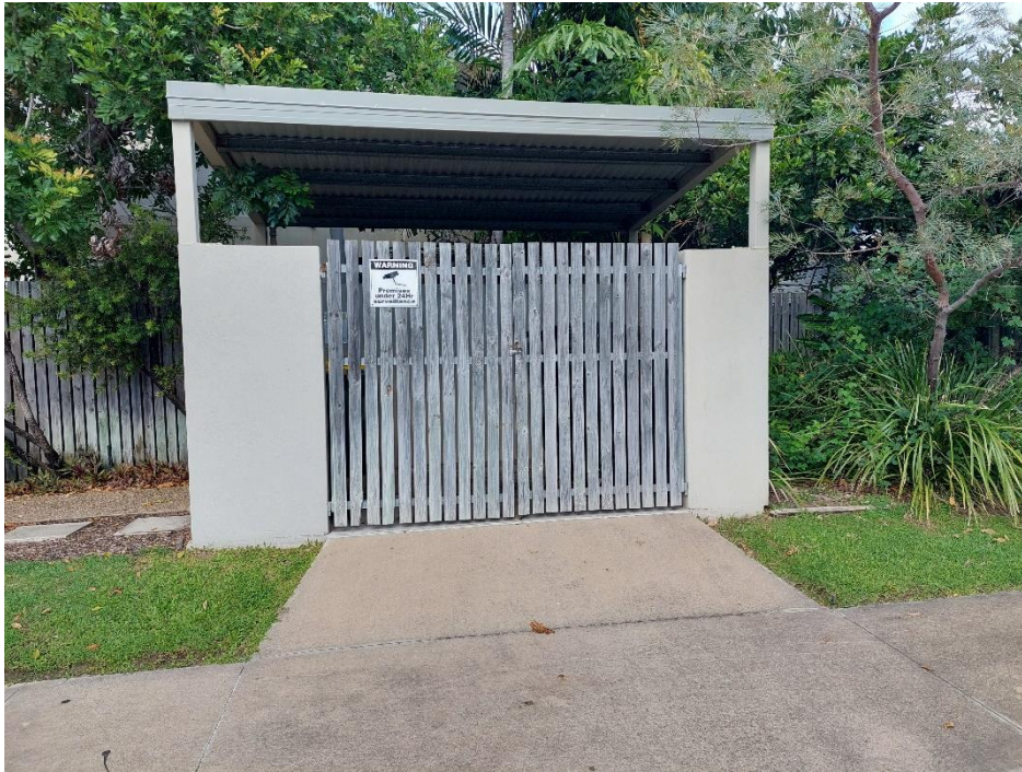
Figure SC6.4.22.2 Enclosed Concrete Hardstand for Bulk Waste and Recycling Mobile Waste Containers
